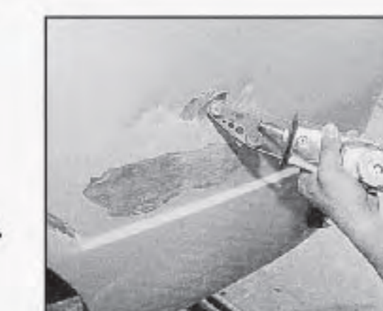
Paint removal work on concave surfaces
